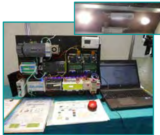
C09. LonMark Japan LON-HDPLC demo. Feasibility test of ANSI /CTA709.8. Controlled ceiling lights (DALI) by commands from MS/TP devices through LONWORKS IP of LON-HDPLC on a single power line.
