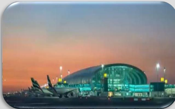
Emergency lighting on large airports e.g. Dubai
